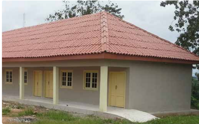
← A school housing project for the Enugu State Education Department in Nigeria, which included construction and renovation works. This image shows one of the lightweight constructions that were clad with Etex ceiling and roofing boards. Picture provided by Emenite.
