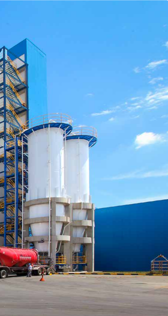
↑ For this Unilever building in Cali, capital of the Valle del Cauca department in Colombia, Promatect H and Promaseal A were used together with Skinco's Superboard. Design: Ingetec S.A. / Installer: SCL Arquitectura.
