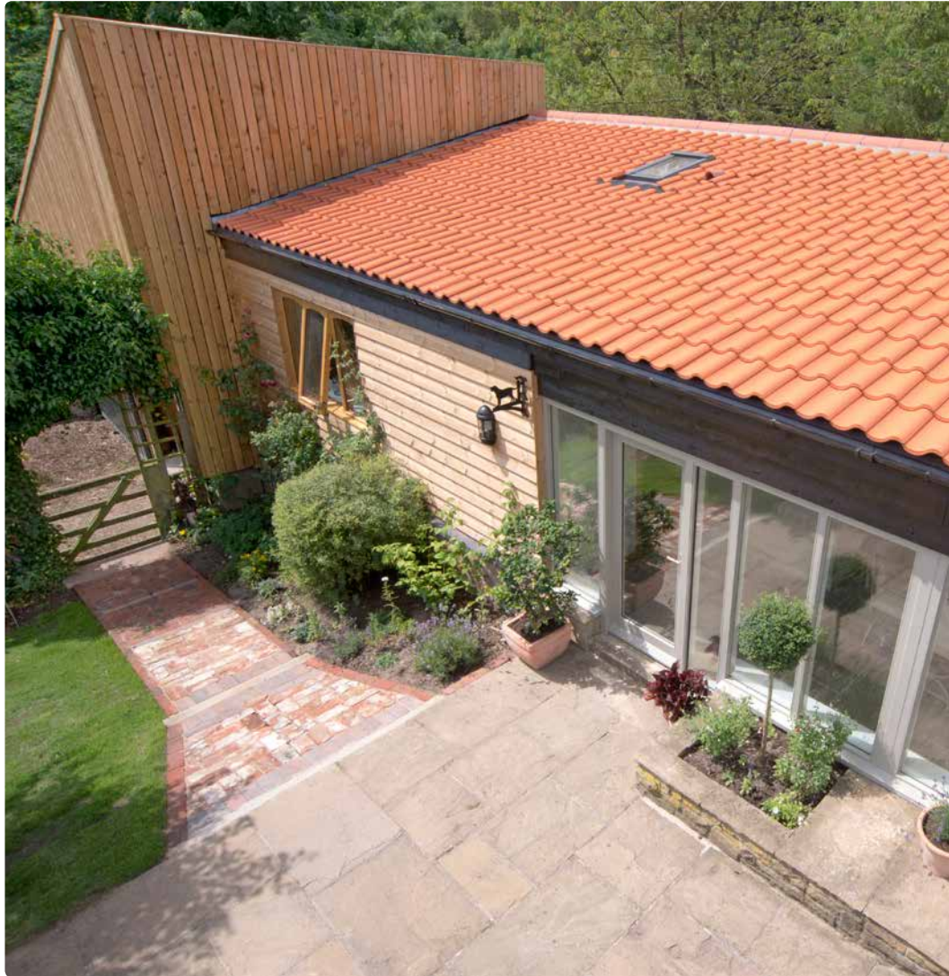
↑ A low pitched barn conversion in Easingwold, North Yorkshire used Melodie clay pantiles in Natural Red to create a stunning guest suite complete with bedroom, ensuite, lounge and kitchen. Architect: Lawrence Hannah. Picture provided by Marley Eternit.
