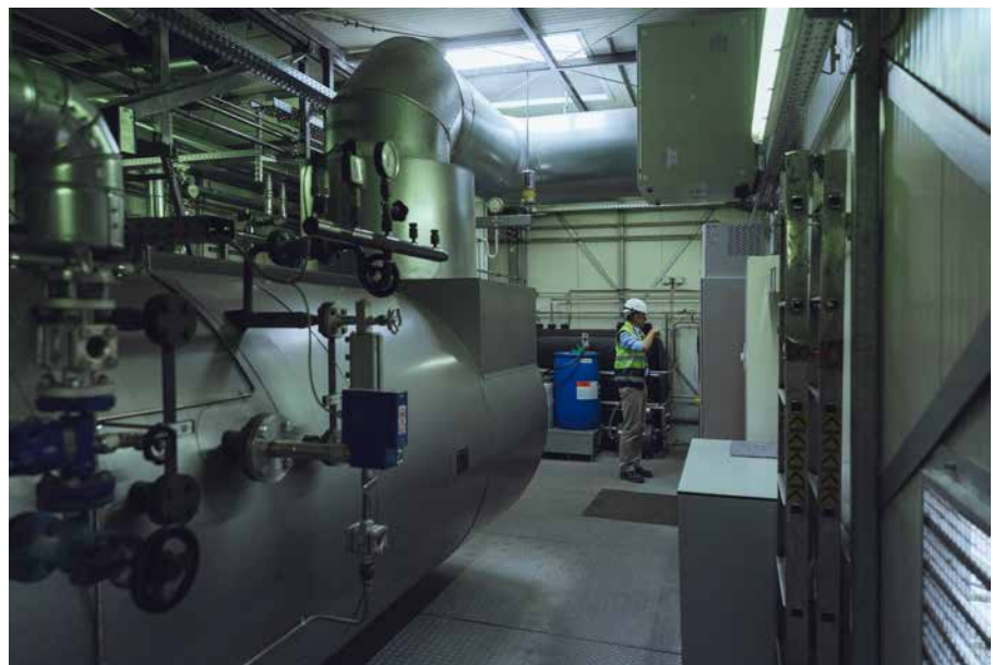
→ At our Eternit factory in Neubeckum (Germany), a cogeneration unit delivers half of the electricity we need. Photographer: Jef Boes, Ghent, Belgium.
