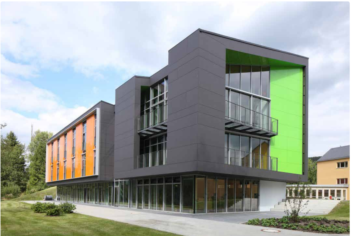
↓ Our black-coloured Equitone Natura covers the Skisport Gymnasium in Klingenthal (Germany). Architect: m2r-architecture, Spitfire Studios, London / Photographer: Conné van d'Grachten, Ulm, Germany.
