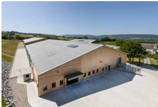
→ Marley Eternit's fibre cement open protected ridges were used to create an effective ventilation system in the bull accommodation unit of this Knocknagael national bull stud farm in Inverness, England, by ensuring a constant outflow of stale, moist air. The width of the air gap created by the open ridge was specifically designed for the number of bulls and size of the building. Contractor: Robinsons Scotland Ltd / Client: Knocknagael Farm. Picture provided by Marley Eternit.
