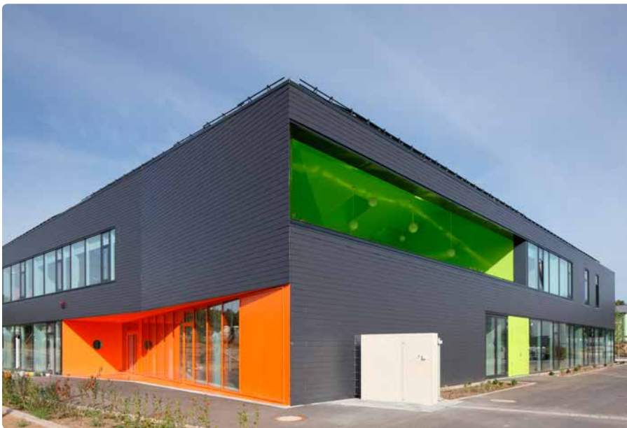
↑ Fibre cement slates on the facade to give this building a sleek modern touch. Architect: Bär, Stadelmann, Stöcker Architekten BDA, Nürnberg. Photographer: Conné van d'Grachten.
