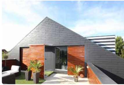
← Blue black fibre cement slates from Eternit Germany are used for this family home in Dieburg, Germany. Architect: Stephan Kollmann, Dieburg. Photographer: Conné van d'Grachten, Ulm, Germany.
