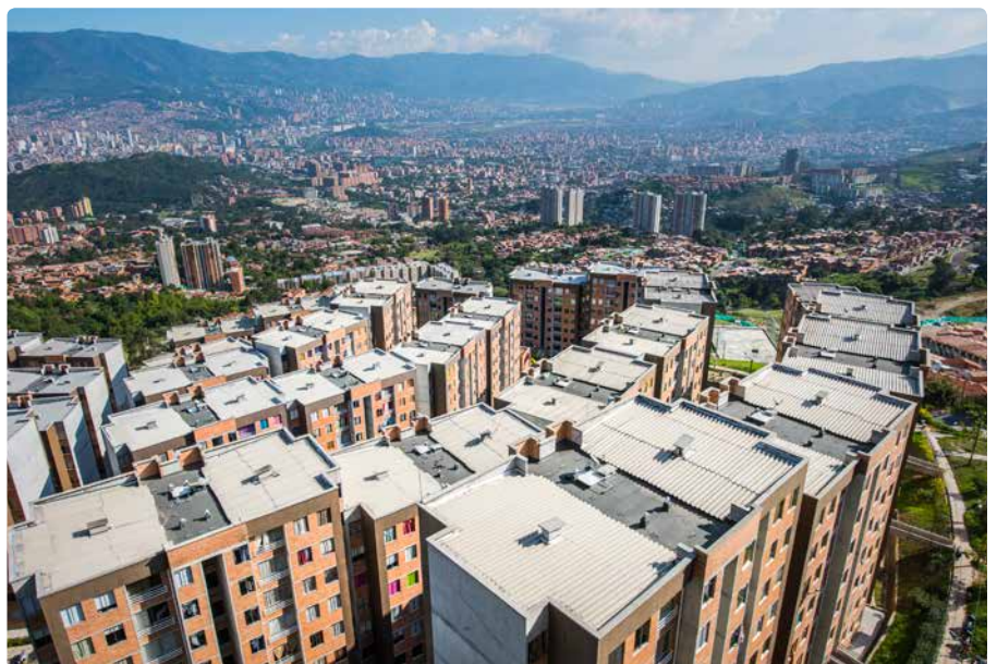
↓ Skinco provided its Teja Superonda for 94 apartments in Robledo, Medellín in Colombia. Constructor: Acierto inmobiliario. Picture provided by Skinco.
