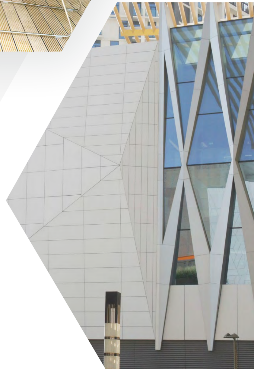
Dubai Expo's metro station featuring EQUITONE [linea] & EQUITONE [tectiva]
