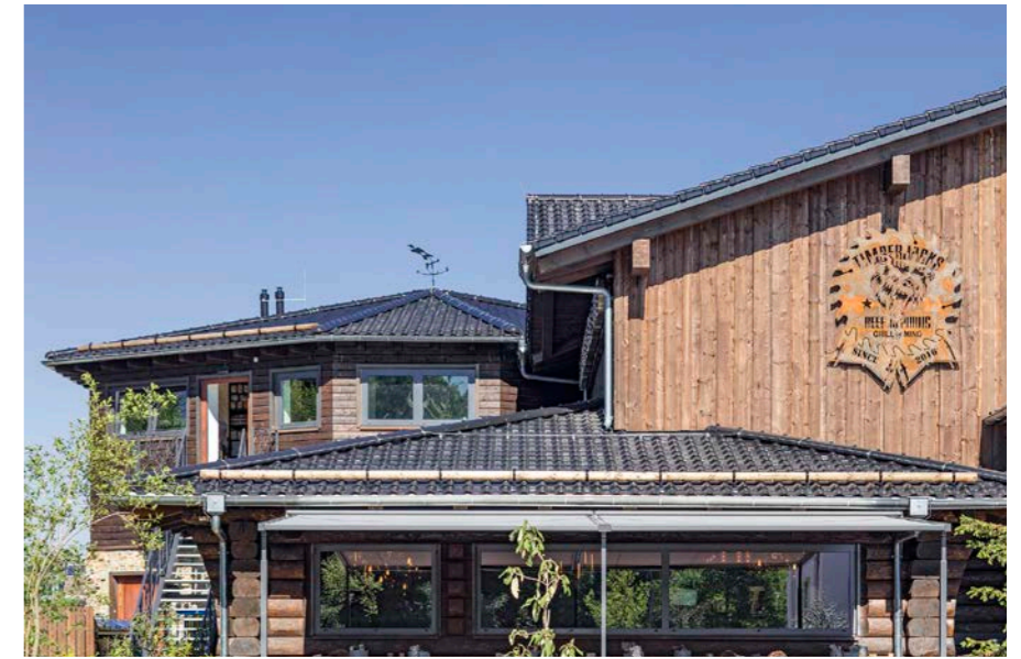
→ To capture a rustic blockhouse style, the Timberjack's Bar & Grill in Göttingen, Germany used Creaton's Futura roof tiles to cover the 1,700 m 2 roof area.
